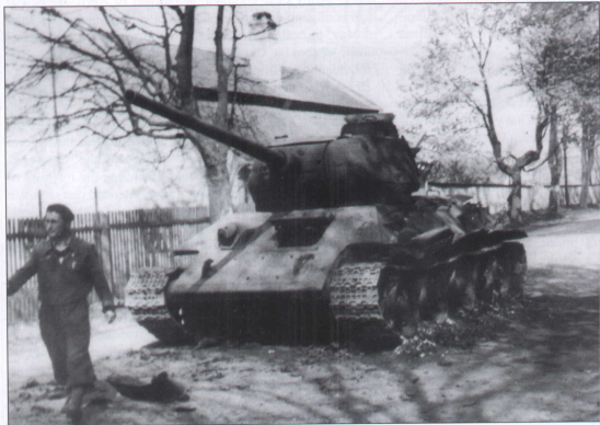
Top: Lt. Gončarenko's tank, detail view. The projectile hit the tur- ret's side, exploded on the house behind the tank and killed tank commander in his hatch.
